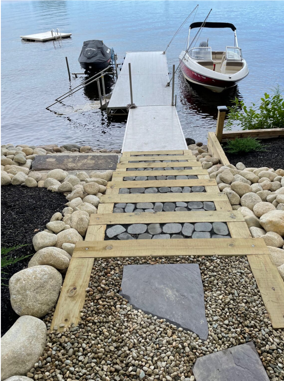
Infiltration steps and stone work for erosion control.
