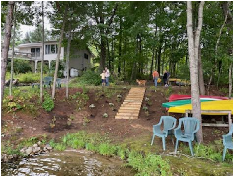
Hi-Vu Road Beach Access Via Infiltration Steps
